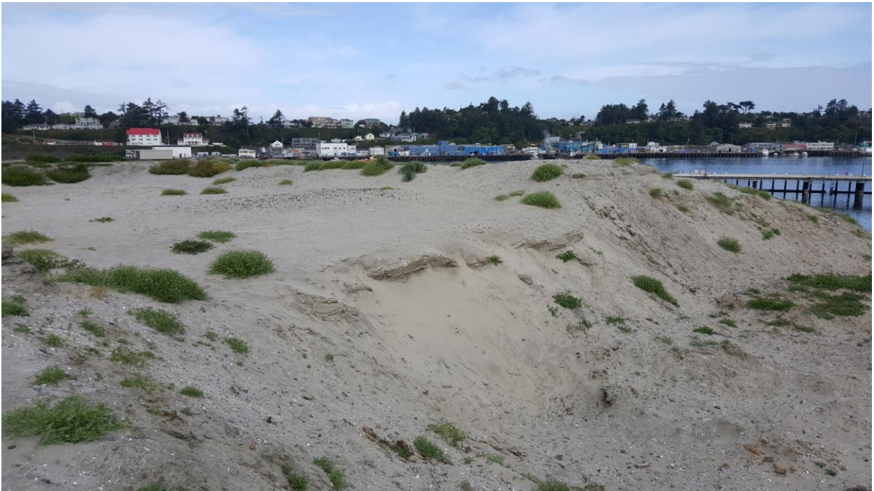
Figure 2 Dredge disposal site looking toward BOAA Pier at the west end
