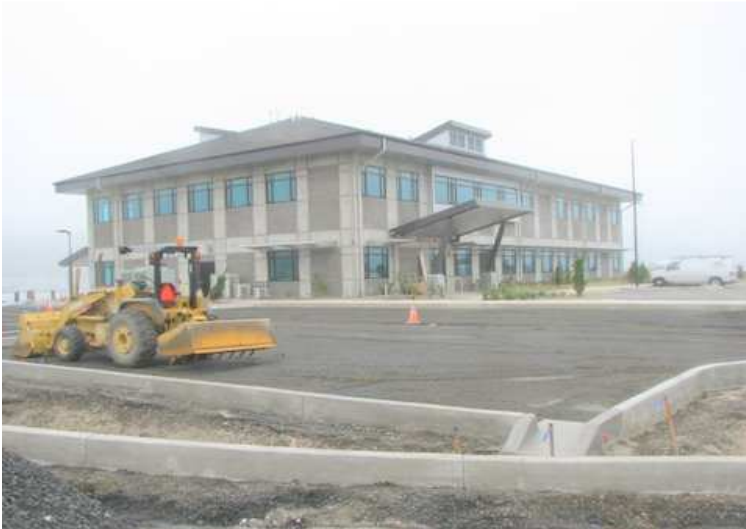
NOAA Administration Building
