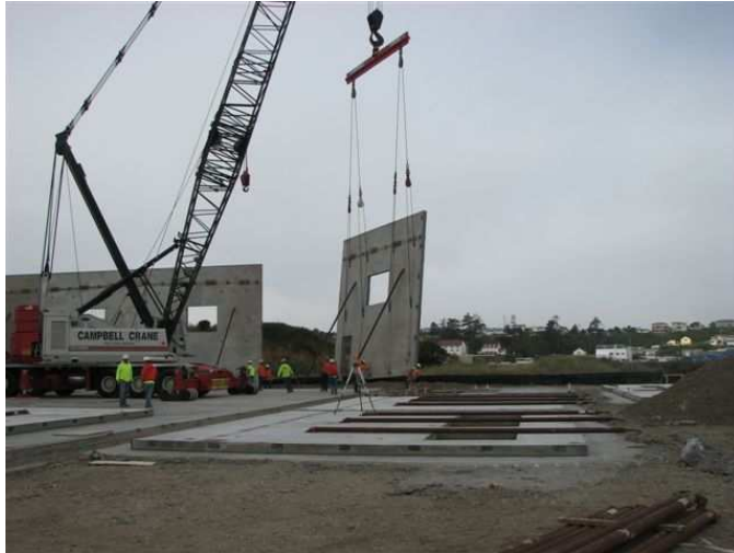
Raising the warehouse walls at the NOAA Homeport site
