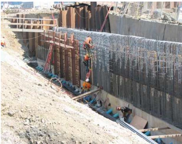
Ironworkers reinforcing the permanent bulkhead wall
