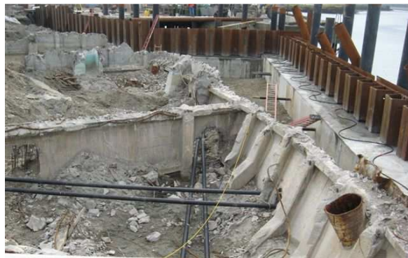
Installation of tension rods through the Hennebique
