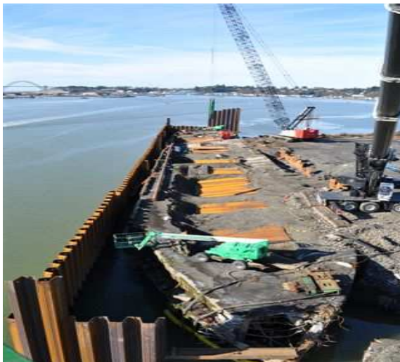
Work in progress on the containment cell
