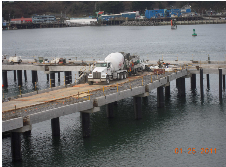
Work in progress on the NOAA pier
