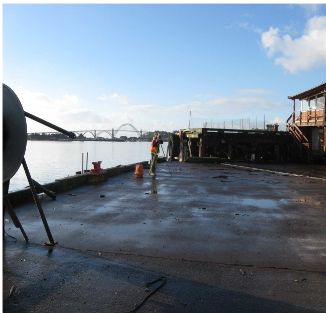
Survey work on the terminal dock.
