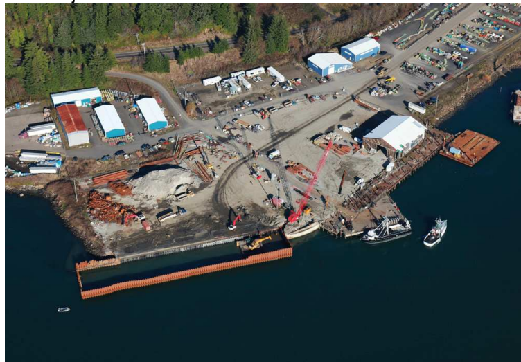
International Terminal Renovation Project December 2011
