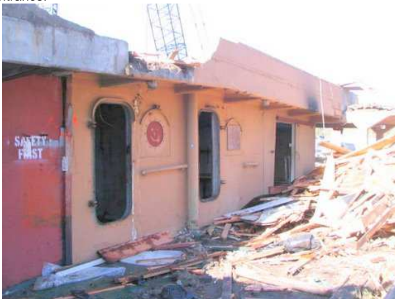
“Safety First” at the old terminal office
