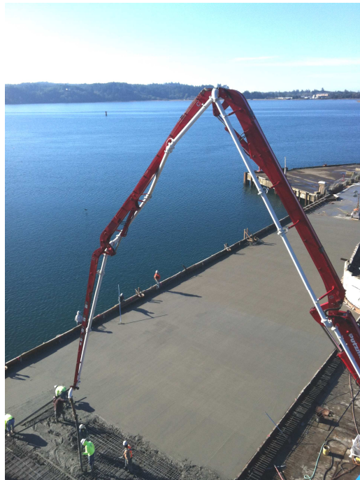
Concrete Pour on the East Dock (Photo by Commissioner JoAnn Barton)
